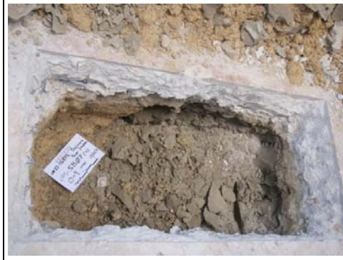
Photo 14. SB07 Hand dug service pit to 0.9m bgl
